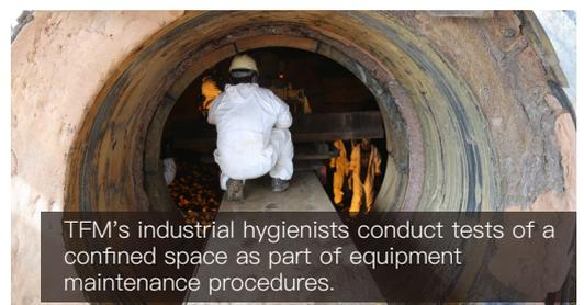
TFM's industrial hygienists conduct tests of a confined space as part of equipment maintenance procedures.
